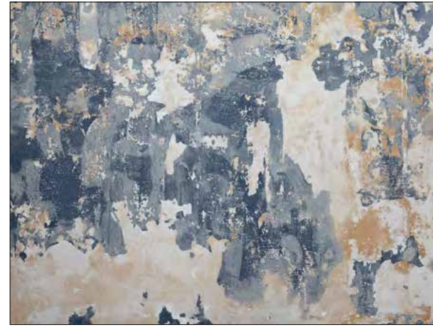
R12791 | BATTERED WALL R
